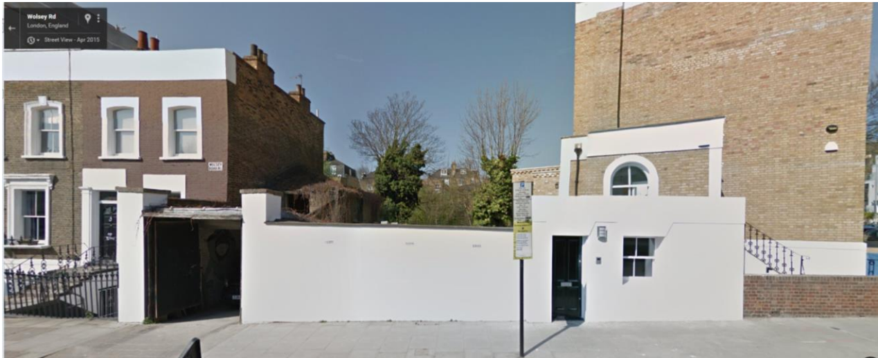
Image 2: Existing Street view of Application Site
