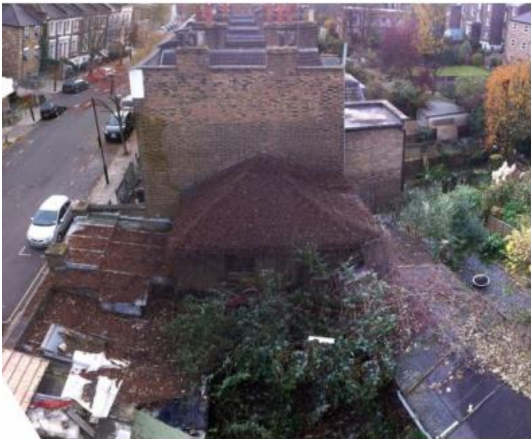
Image 4: View from the rear of 121 Mildmay Road.
